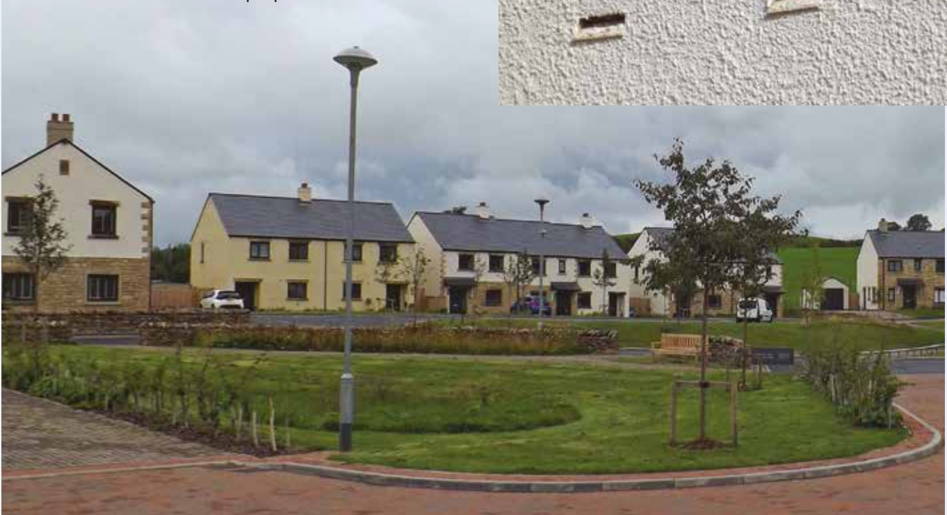
Main image: Rawthey Meadows, looking west Above: Bat boxes
