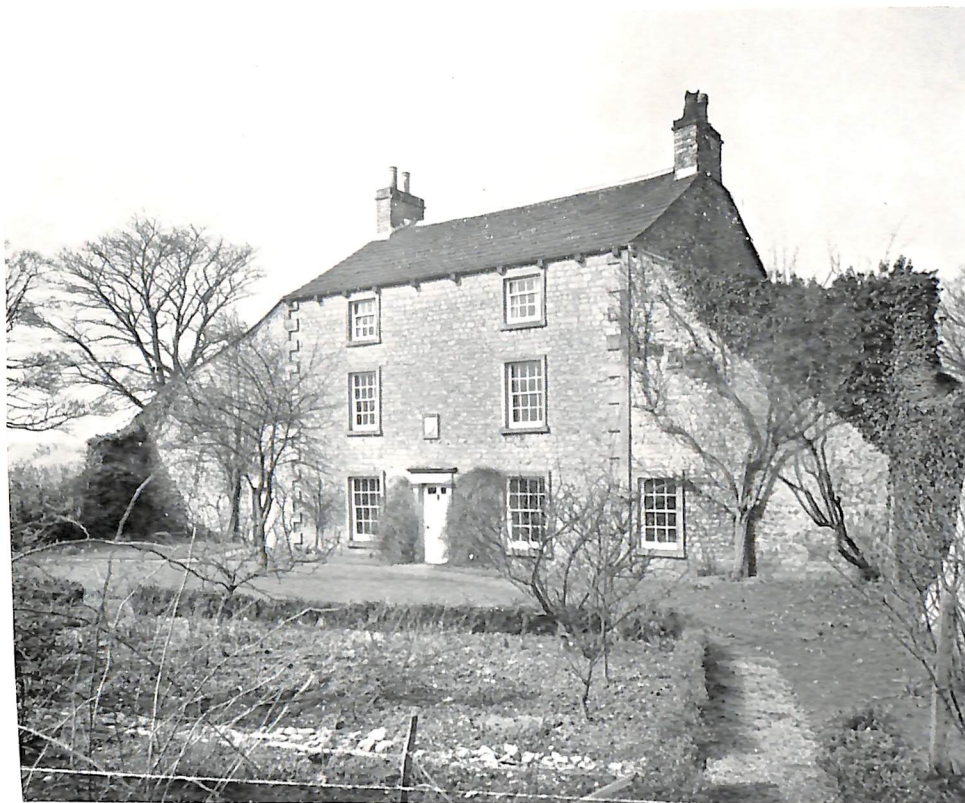
Eshton Grange Farmhouse (Lot 3)
