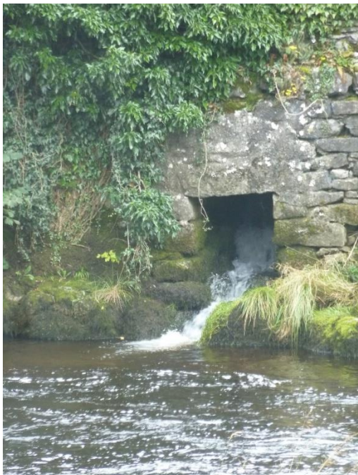
Water outlet, Settle Bridge
