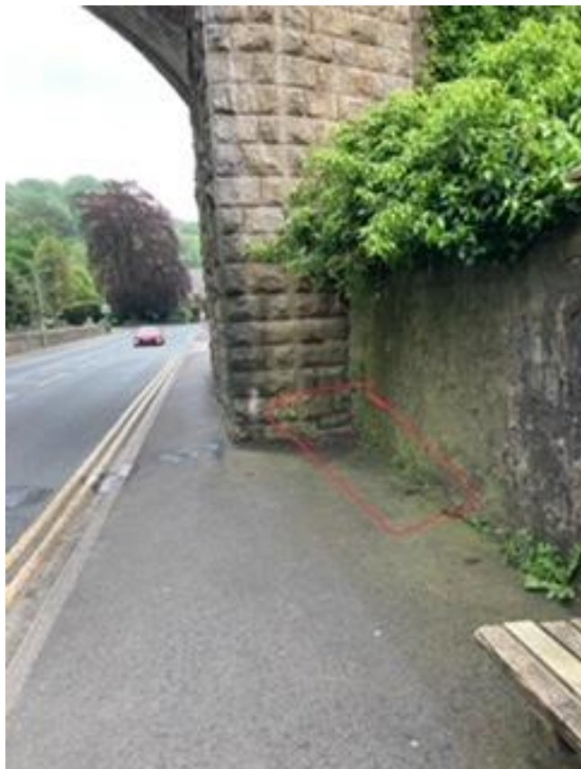
Trough site under railway bridge on Church St
