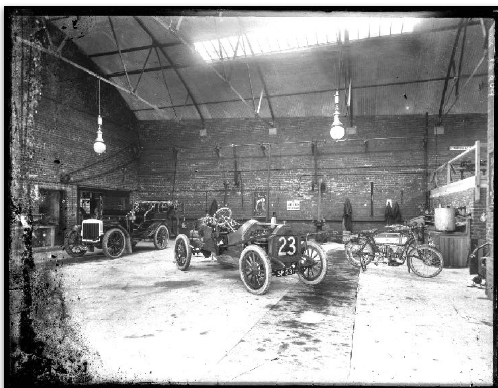
Ellis garage interior, photograph by the Horner Studio. Horner Collection©NCBPT (CC-BY 4.0)
