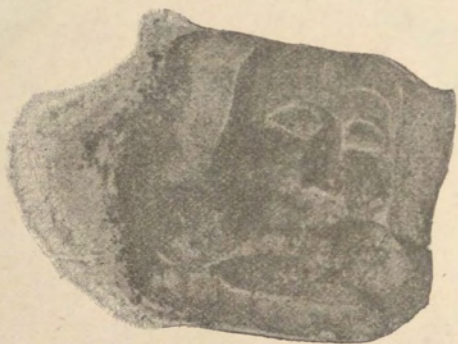
Stone Corbel in Giggleswick Church.
