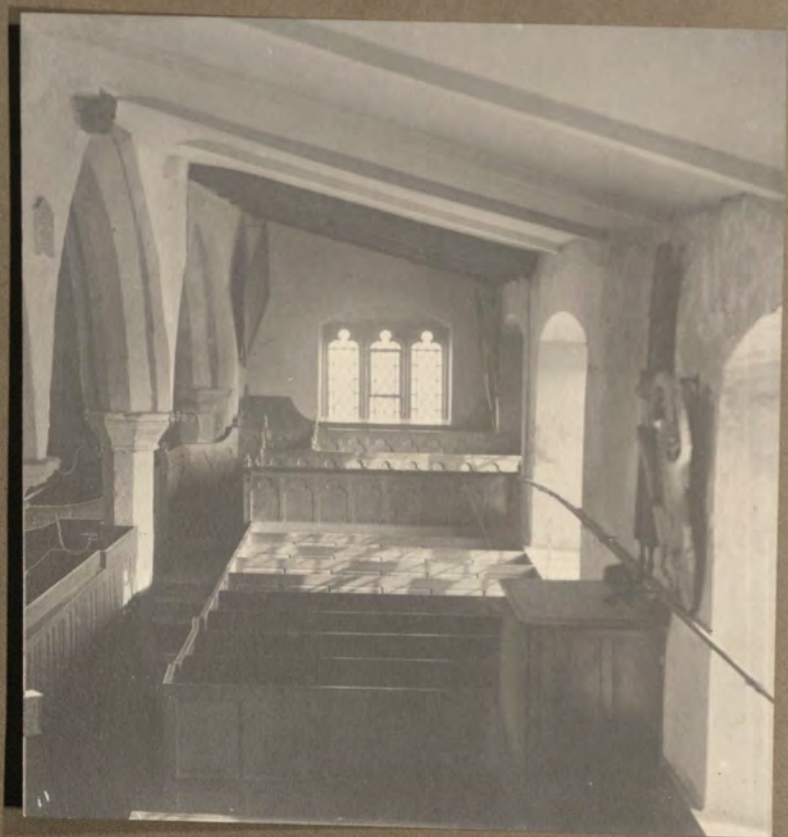
East end of South Aisle prior to the restoration.
