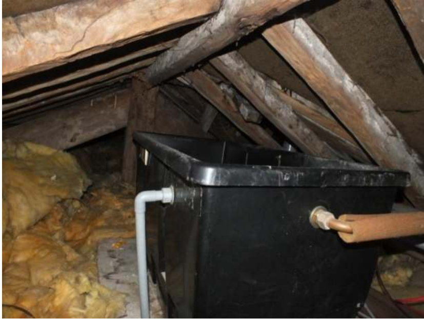
17thC kingpost roof truss
