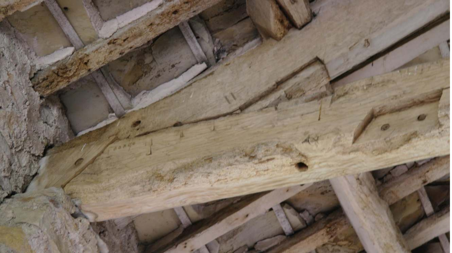
Truss 2. Cruck blades c1540 re-used as principal rafters and tie beams
