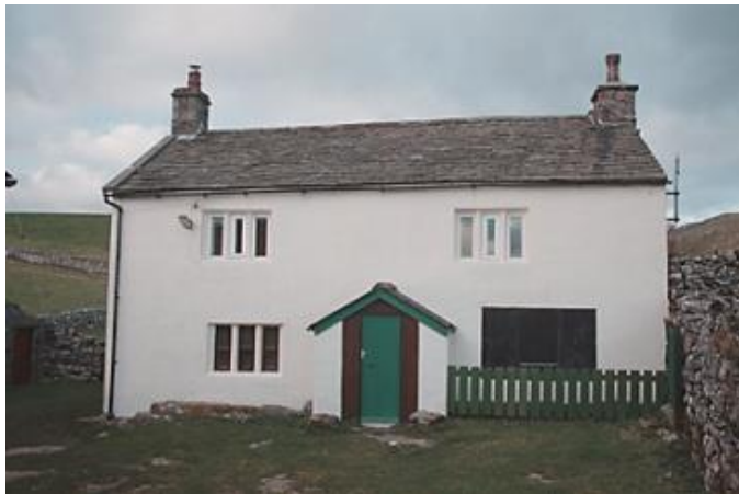
House built c1720
