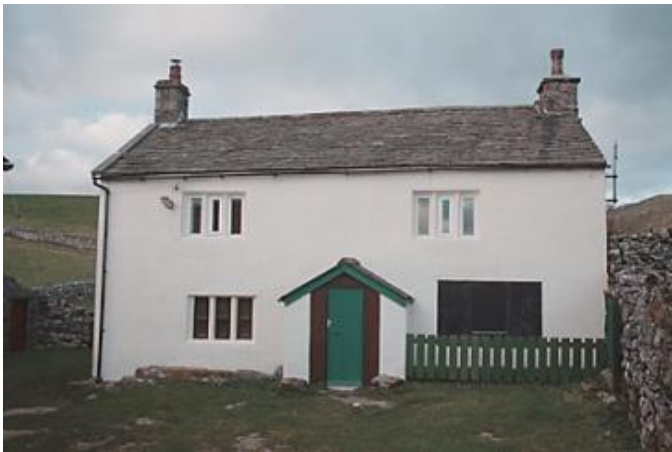
House built c1720
