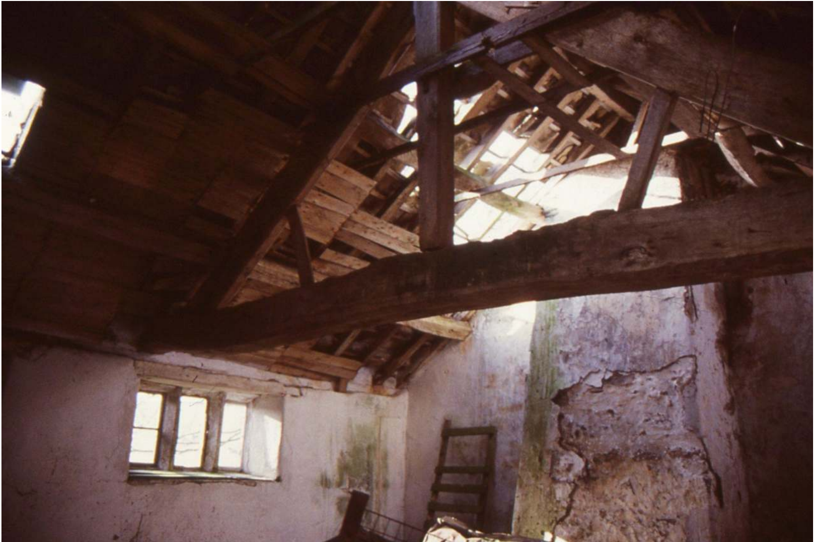
Kingpost roof truss 17thC (firehood in background)
