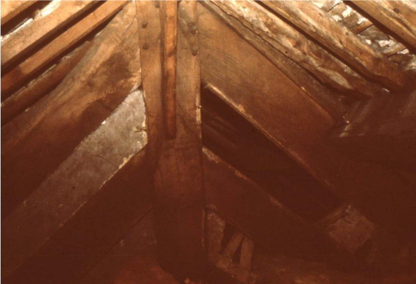
c1500, Addingham Kingpost truss with A-framing
