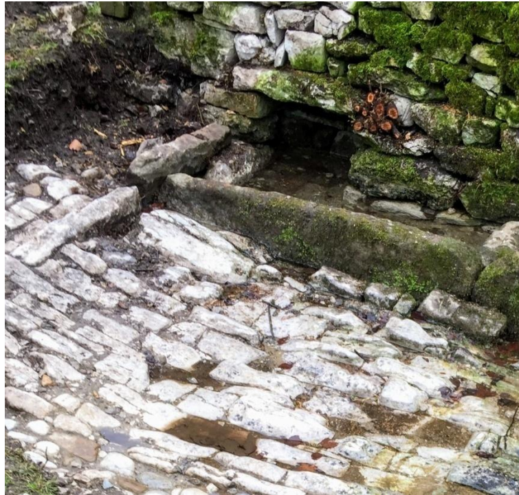
Photo 6 Trough 1 after clearance.
