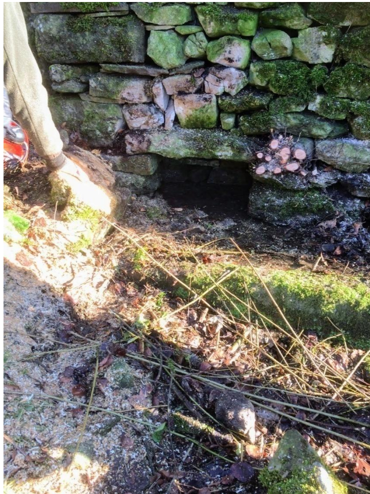
Photo 5 Trough 1 before removal of sediment.
