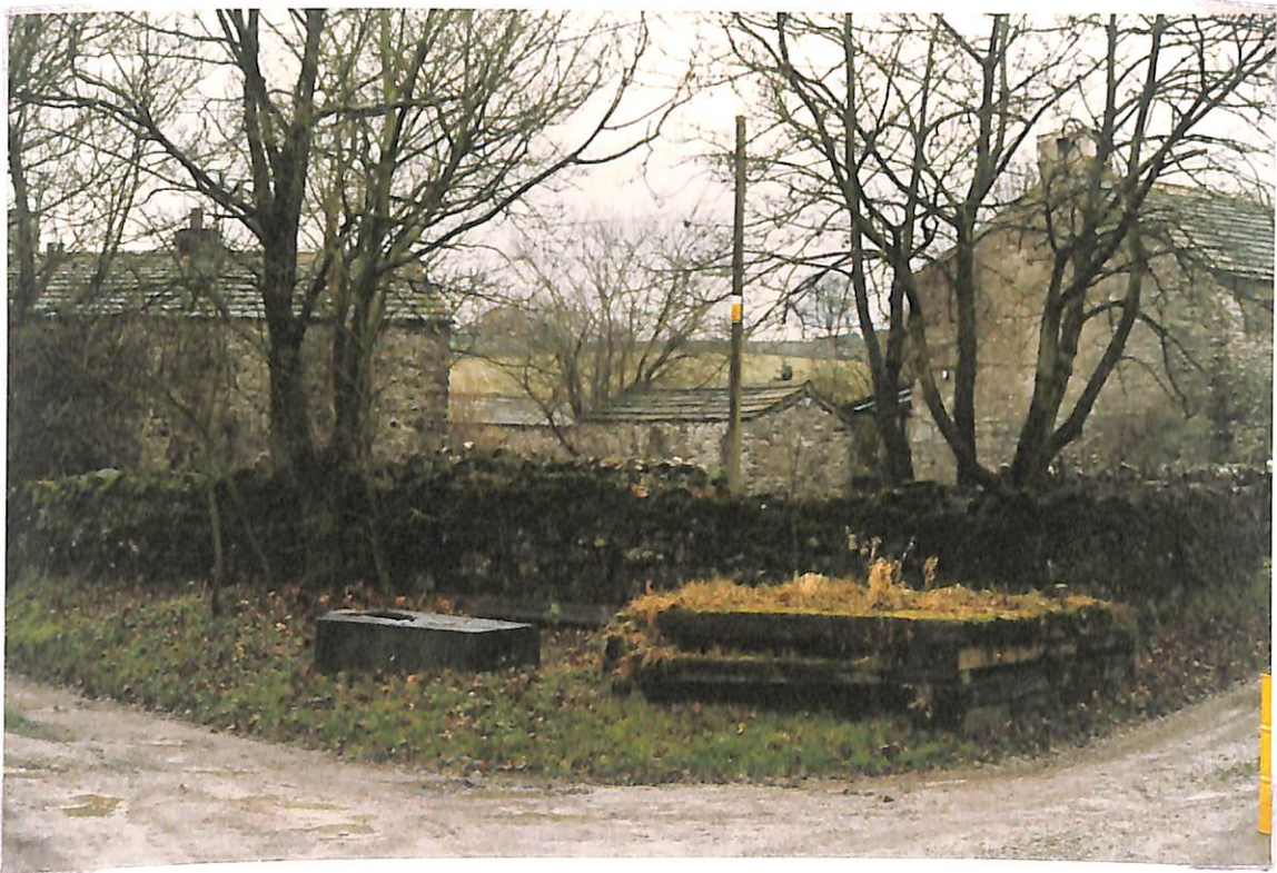
1998, before clearing tank and sleepers.
