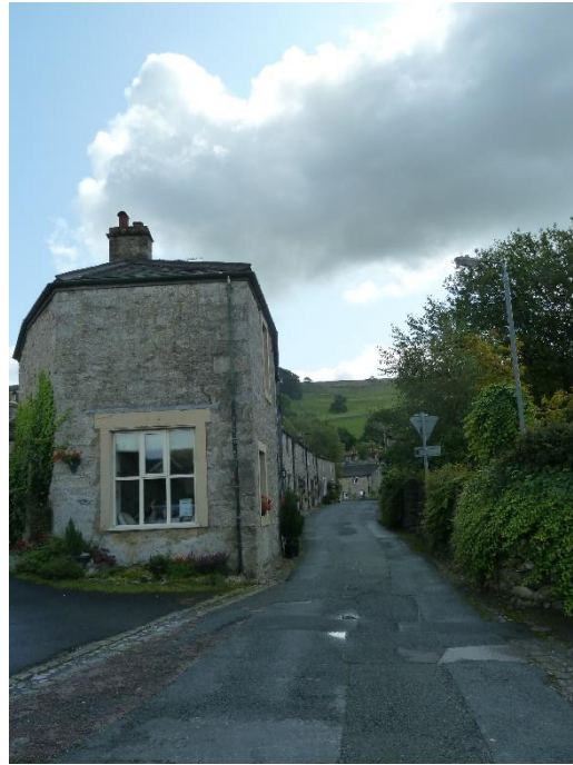
Figure 3 New Street Stainforth Road end showing no.11
