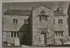
Fig. 1: Old Manor House, Clapham. Former Manor House, now backhouse, cleft and bar. Dated 1701 over doorway and on fireplace, with early twentieth century alterations to left-hand doorway. Walling material is rubble, mainly limestone, with sandstone dressings. Roof has been raised by about 18". Described in the Peasner guide (2009) as being richly detailed, although quite small. Porch has dovetail in triangular arrangement giving a pleasing appearance, which could mean that it was for display, as dovetails can be used in the attic of the main house. Nearby houses with similar dovetails are: Three Head Farm, Nearby Manor House at Wurts, Austwick, and Southam Hall. All windows at the front are oval-headed, elsewhere straight chamfered, sometimes with only a slate drip-mould. The stepped drip-mould above the porch window also has spiral steps and a small triangle or 'gable' rising from the centre. Entry is into the right-hand room. Most interior arrangements have gone.
