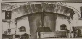
Fig. 4: Old Manor House. Arched fireplace. Mantel square, half-arch fireplace with 16 joggled masonry with ornamental legions, all springing from impost blocks. Two broad ovals.
