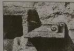
Fig. 3: Old Manor House, decorative drip-mould step. Very unusual mixed, knob-like drip-mould step above basement window, not known elsewhere. There is another one over the round-arched single-light window in the gable wall which faces the road.
