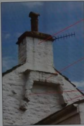
Modern stack Old fire smoke box Corbel ends
