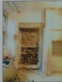
Old blocked doorway
