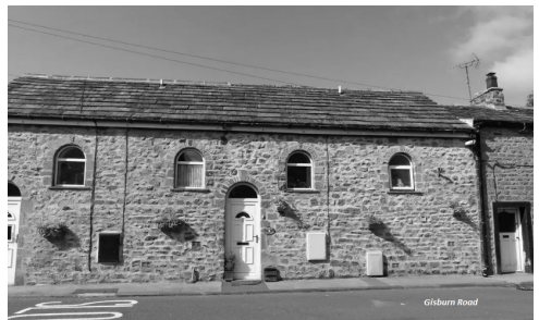
Present day view of the Gisburn Road gasworks
