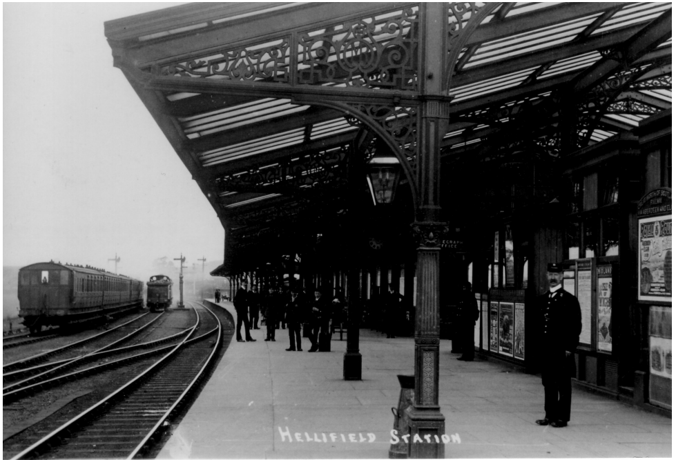
Albert Straw on Hellifield Station
