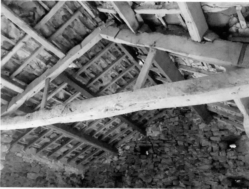
Figure 2a/b: General views of the trusses
