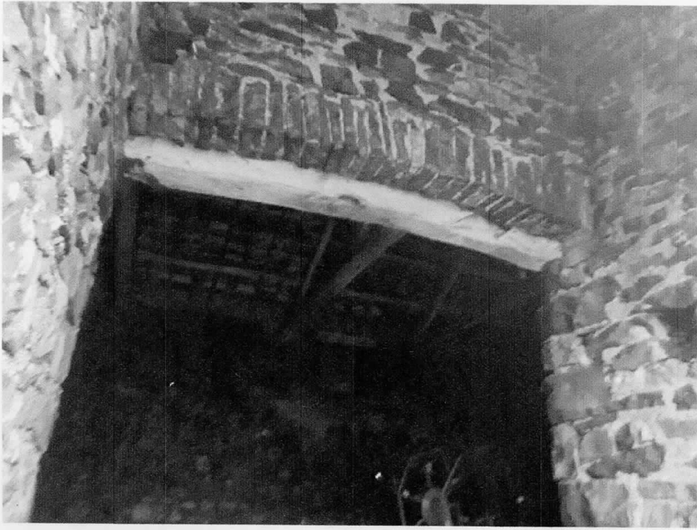
Figure 3: General view of the doorway lintel
