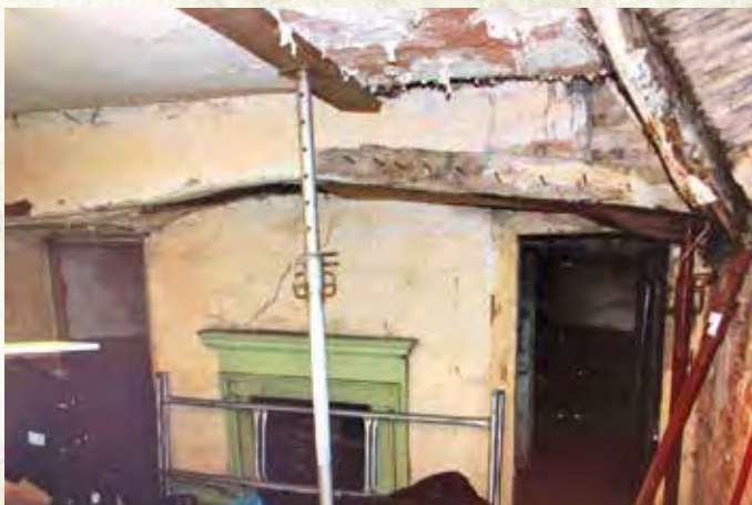
South Carr Farm, before insulation and lime plaster
