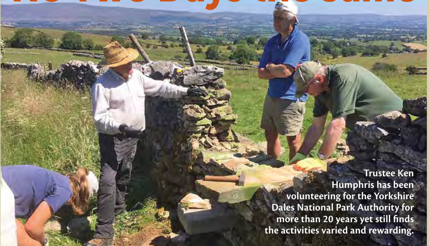
Dales volunteers repairing a stone step stile above Crosby Garrett, looking out over the north Pennines.
