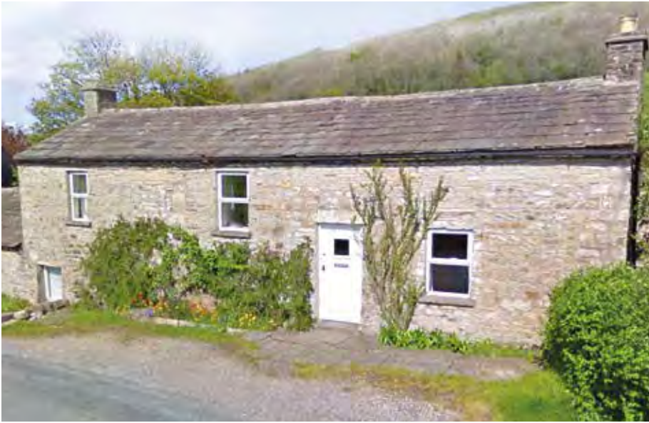
The Bungalow, front view.
