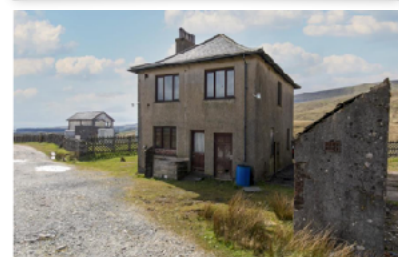
3 Blea Moor Cottages, Ribbleshead, Chapel-le-Dale @ Seorrap
