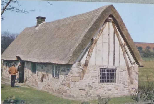
Cruck construction with two angled timbers
