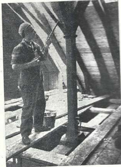
Spraying a king-post with insecticide.
