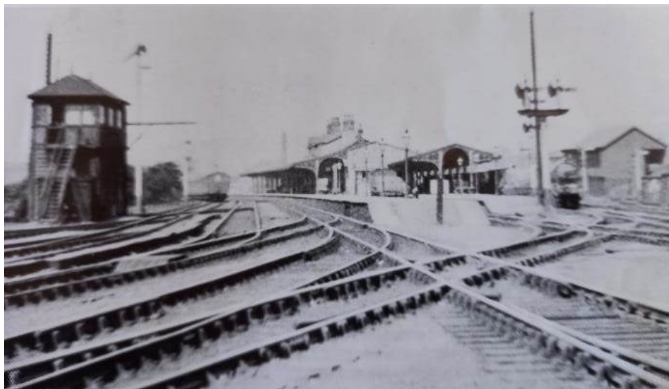
An interesting view of the Station prior to 1911, when the Signal Box was located on the other side of the tracks to where it stands now.
