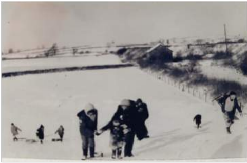
Back up the hill alongside Dunbars. Interesting photo as it shows the Midland Railway Pumphouse still in situ. 1968.
