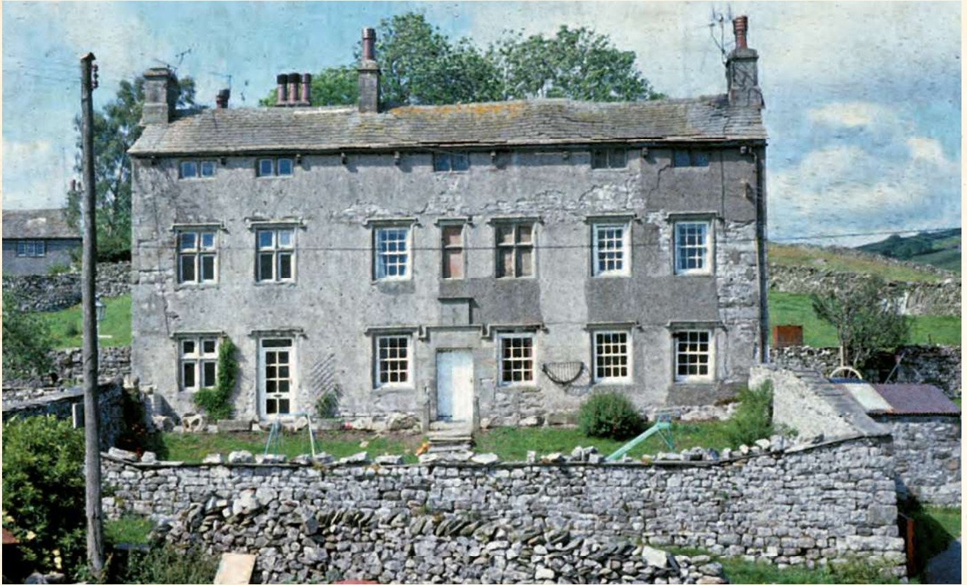
When photographed in 1974, Knight Stainforth Hall had the remains of a lime render, patched with cement. Its removal led to years of damp problems. Photo courtesy of Jonathan Ratter
