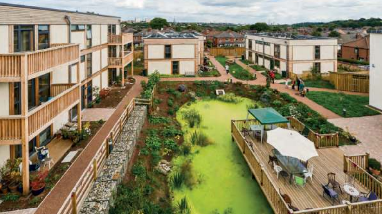
Views of Lilac Grove cohousing project. Photo courtesy of the LILAC project
