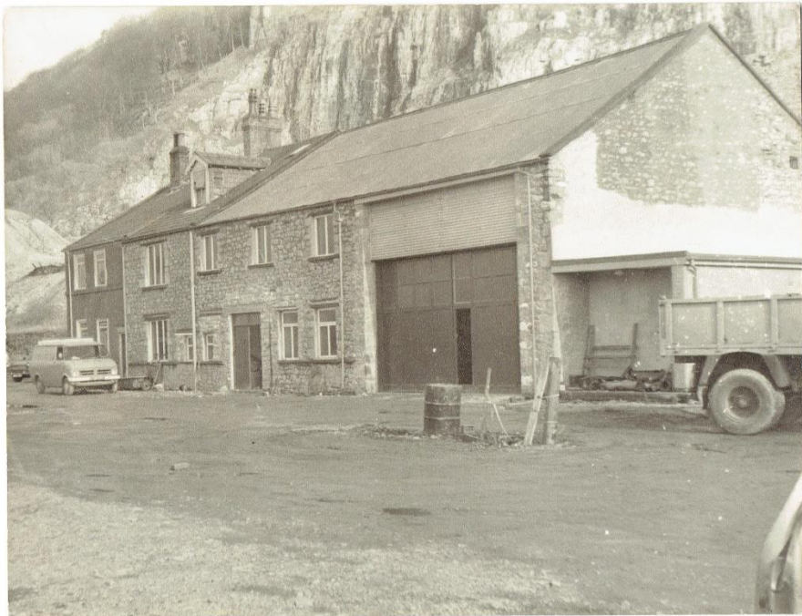
MAIN BUILDING 1/2 COTTAGE, WORKSHOPS, GARAGE WORKSHOP
