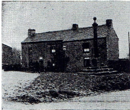
The old post office at Austwick, long since demolished. The Calverley family were associated with the Royal Mail for many years.
