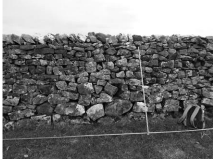
FIGURE 1 A typical Langcliffe wall showing 1.5m measuring stick and tape base-line
