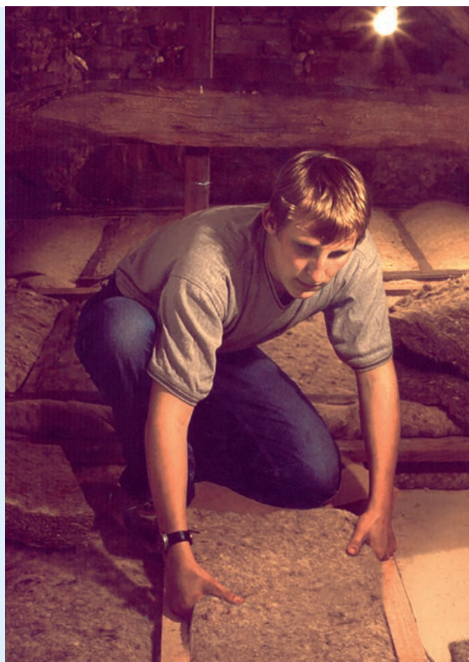
Installing Sheep Wool insulation
