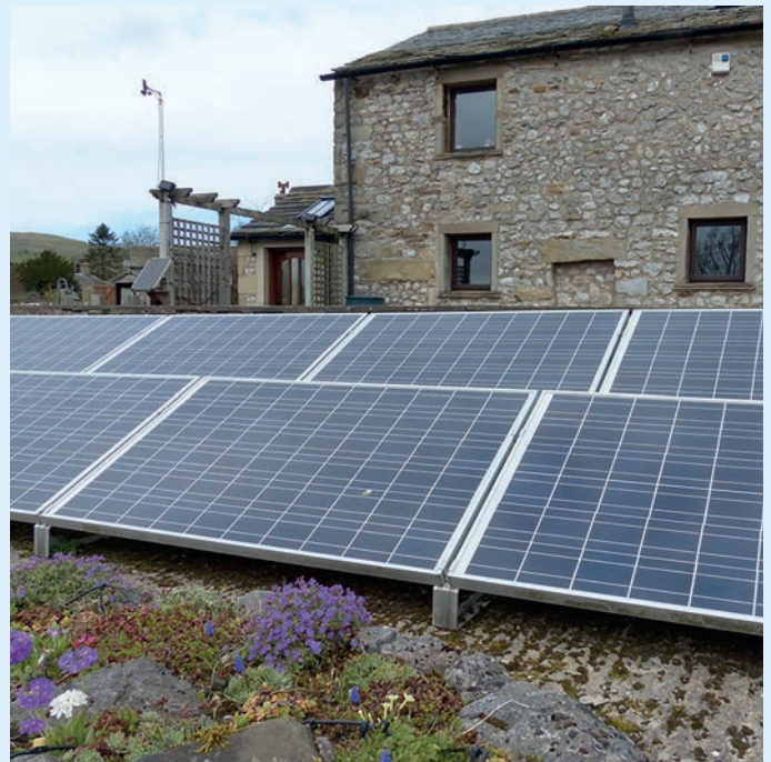
Solar Panels in Malham garden
