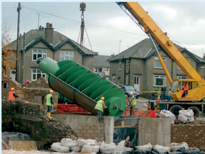
Installing the Settle Hydro
