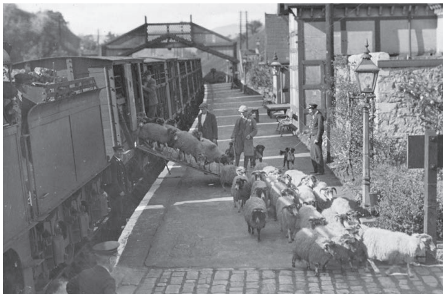
Livestock and freight unloaded in earlier days
