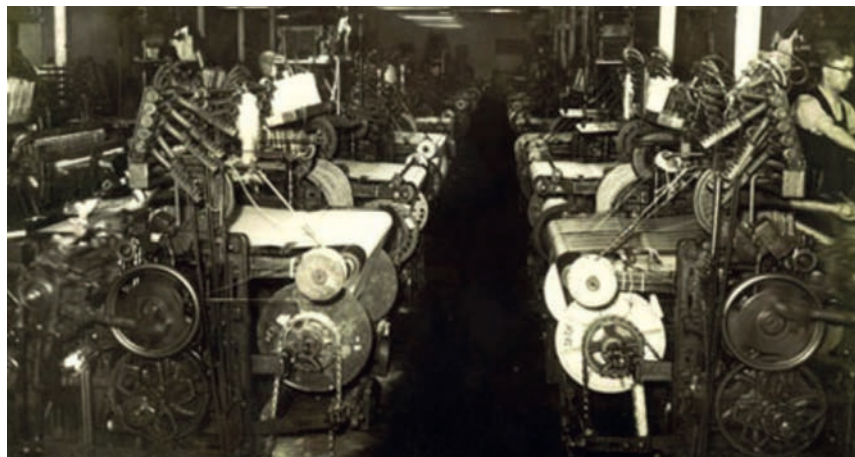
Skipton Mill circa 1959 with Lancashire style non-automatic circular box made by Hattersley of Keighley. They produced high class dress and umbrella fabrics from man-made fibre yarns. Photo by kind permission of Mrs C. Todd.
