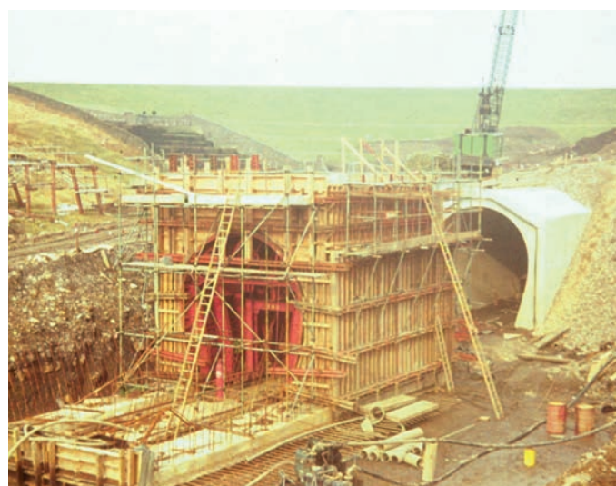
Outlet tunnel construction
