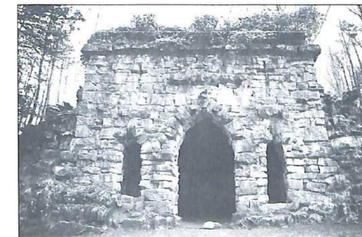
The photograph of the grotto on the Ingleborough Estate (above) and the drawing of the field lime kiln in operation (left) are taken from the book 'Heritage on Foot', reviewed on page 14, opposite.
