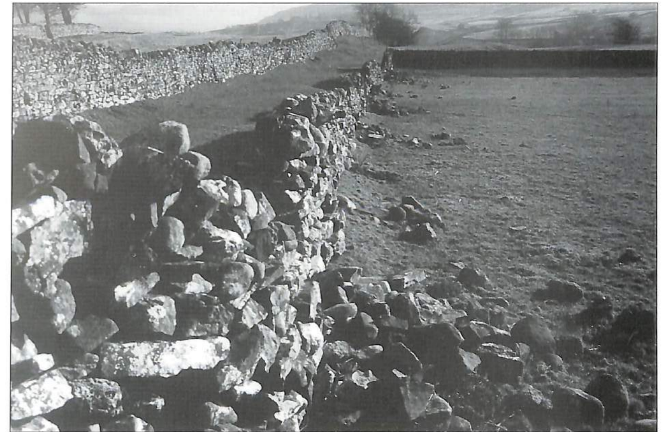
3. Dereliction of dry stone walls in the Dales is an increasing problem due to changes in farming practices over the last few decades. Stretches like this one at Grassington will be restored over the next four years. The first year's projects are being assessed at the moment and should result in around 6km of these key landscape features being restored with a further 22km by the end of the project.
