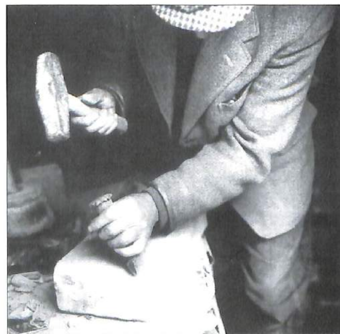
Photo: Pitting off the rough stone with a pitting tool – from the book "Making Stonework" by Marie Hartley and Joan Ingilby.
