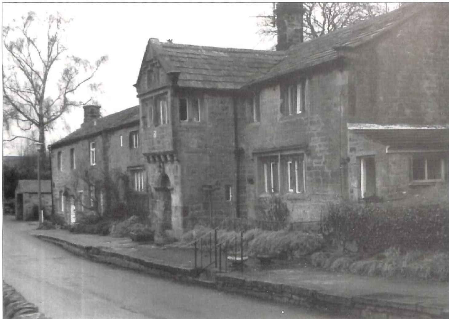
17th Century house at Embsay. Note the hood mould, the coping and kneelers and the superb porch with typical three-light window in the gable.
