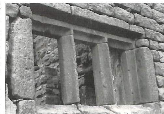
Convex mullions at Gate Up - a long abandoned house at Grimwith.
