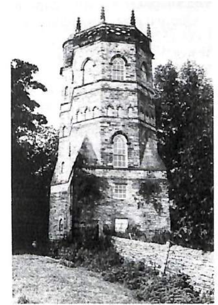
The Culloden Tower, Richmond
