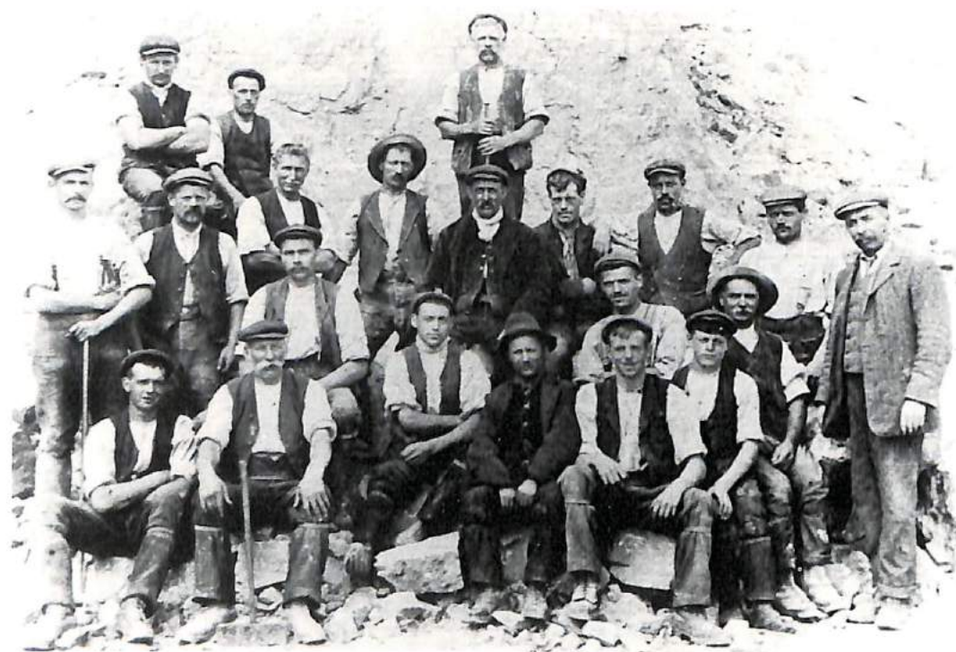
No photograph of navvies building the Settle-Carlisle line survives. However, these Yorkshire quarrymen from the 1880s include men who stayed on after the line was completed
