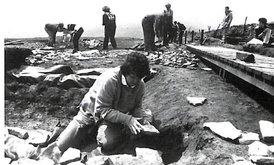
Siltraps and boardwalk construction, Pen-y-ghent (Photo Alan Atkinson)
