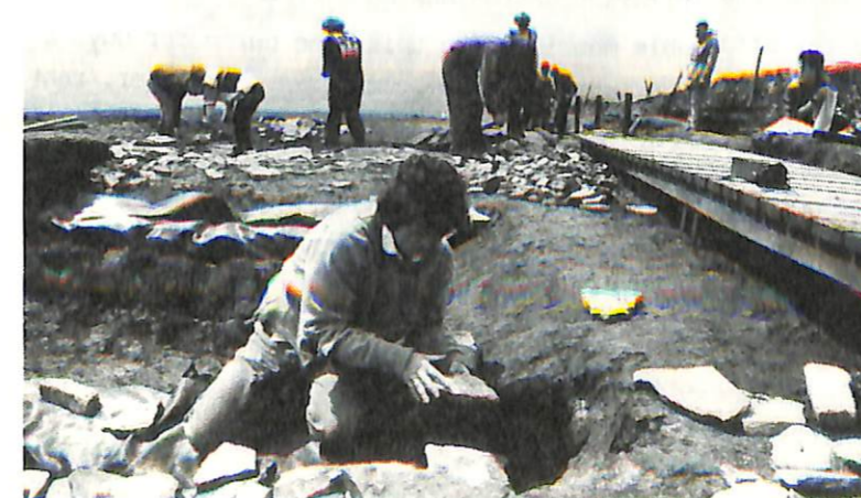
Silttraps and Boardwalk construction, Pen y Ghent (Photo: Alan Atkinson)
