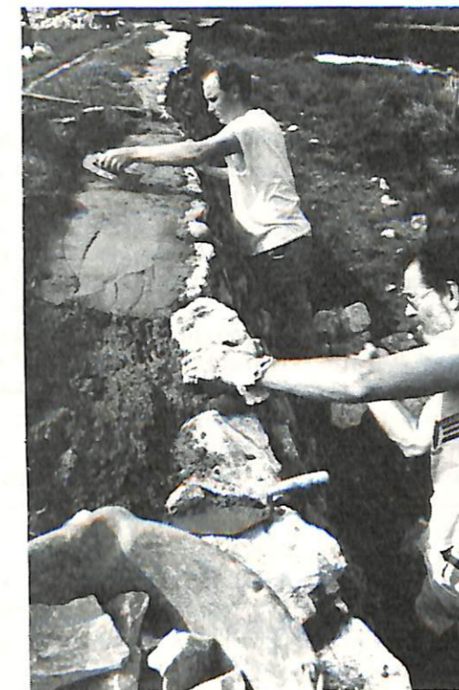
Revetting the Dalesway Footpath, Wharfedale (Photo: Alan Atkinson)
