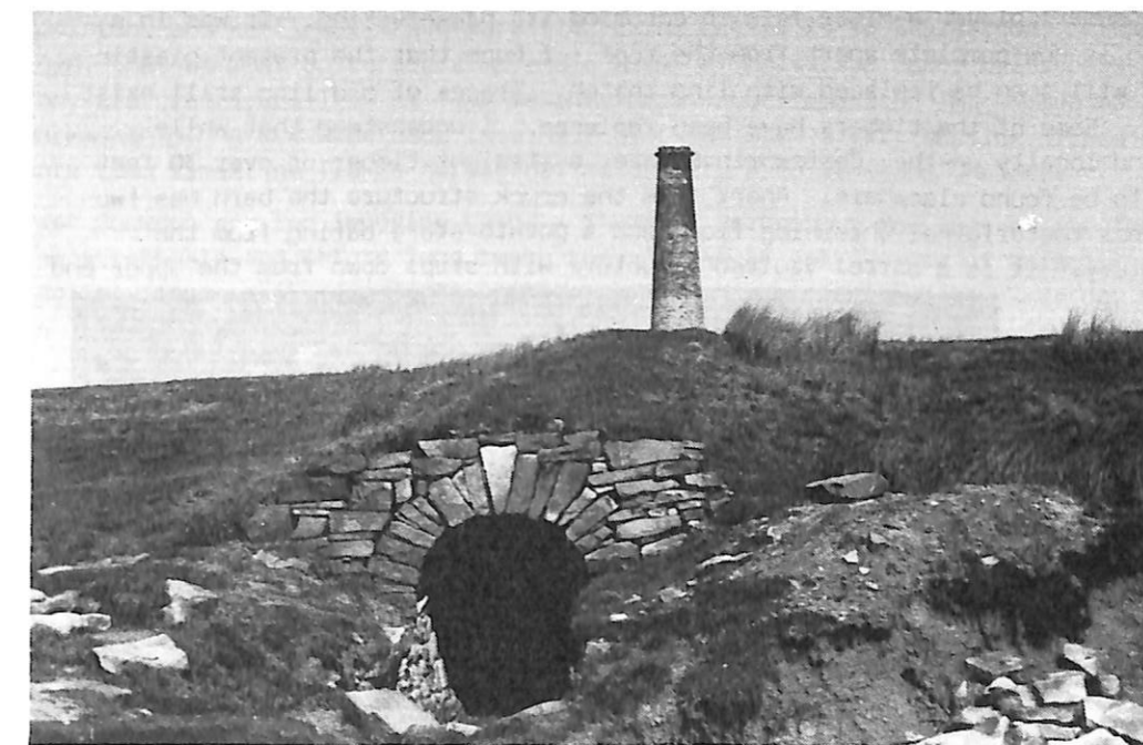
The flu system and smelt mill chimney, Grassington Moor.
