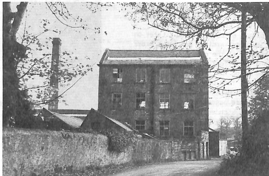
Linton Mill, Upper Wharfedale - a 19th century textile mill with a medieval watercourse, demolished in 1984 for housing development
