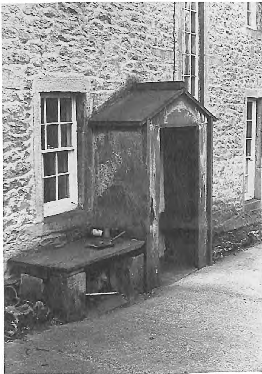
FIG. 5. A porch of high quality workmanship. The use of Flag extends to ledges within the porch. The farm is near Settle, in North Ribblesdale.
