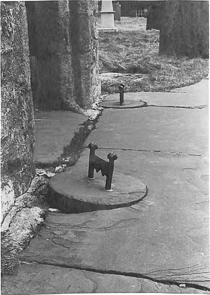
FIG. 12. Horton-in-Ribblesdale Church. The path and circular base of the foot scrapers are composed of Flag.
