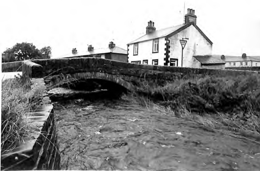
Horton Bridge near Burnside.
