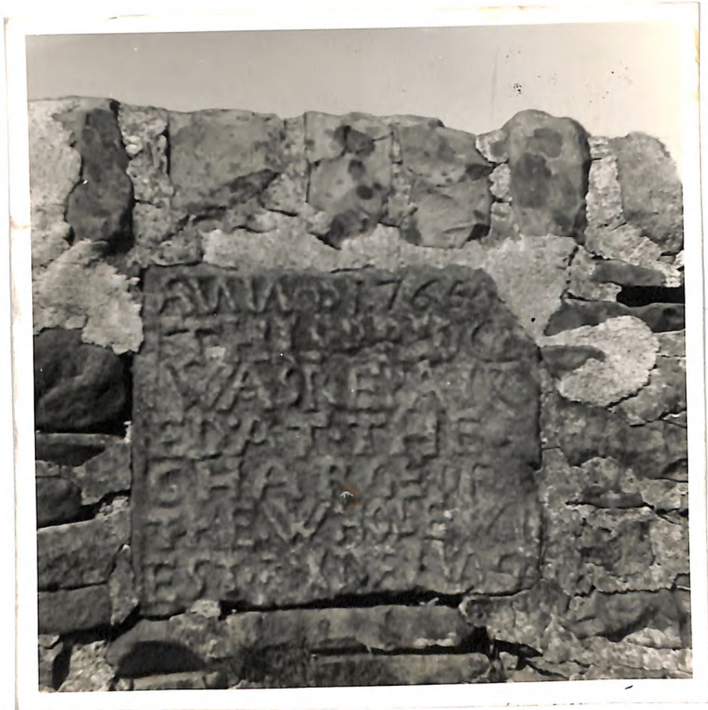
Ling Gill Bridge.
