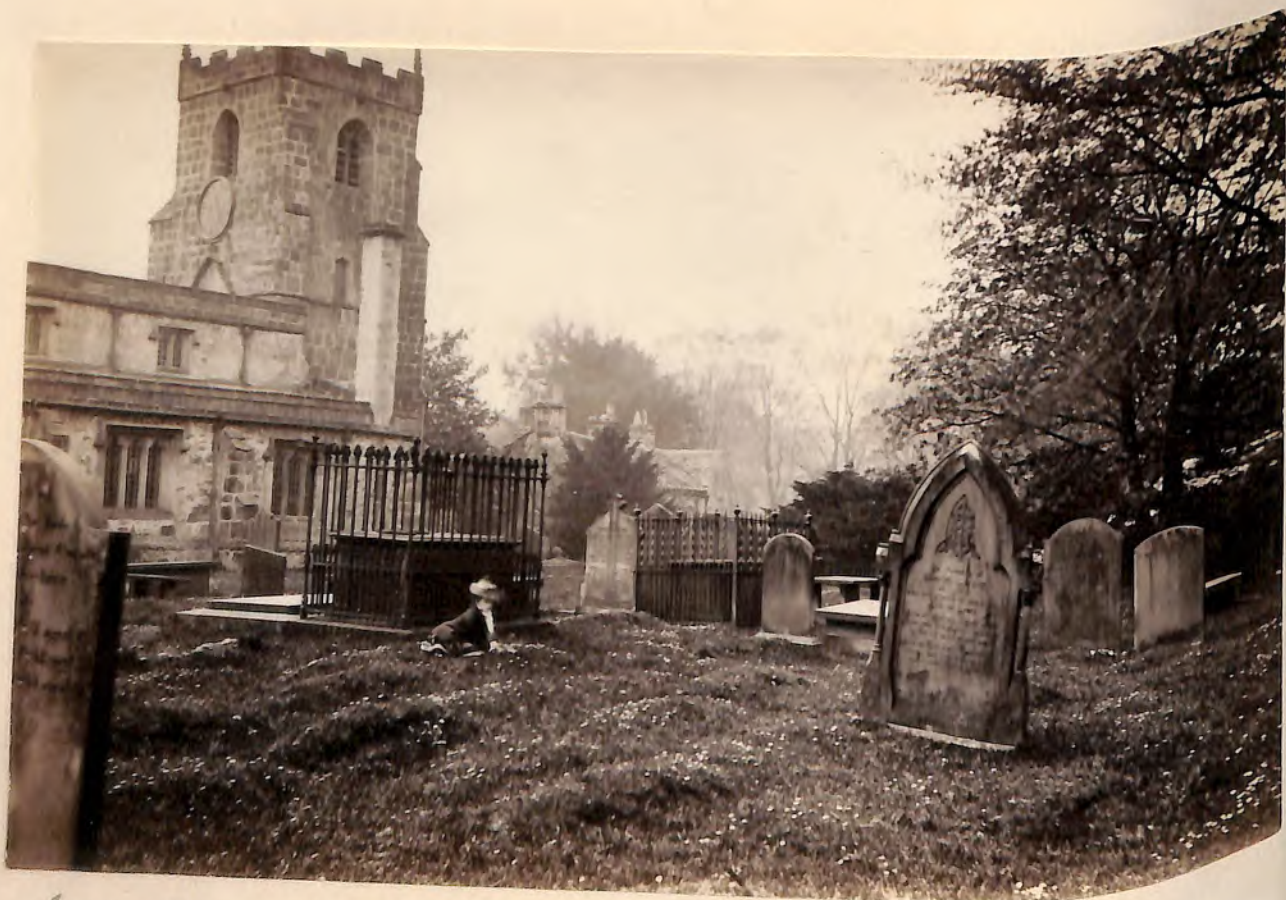
Note Chimney of old heating-furnace.
