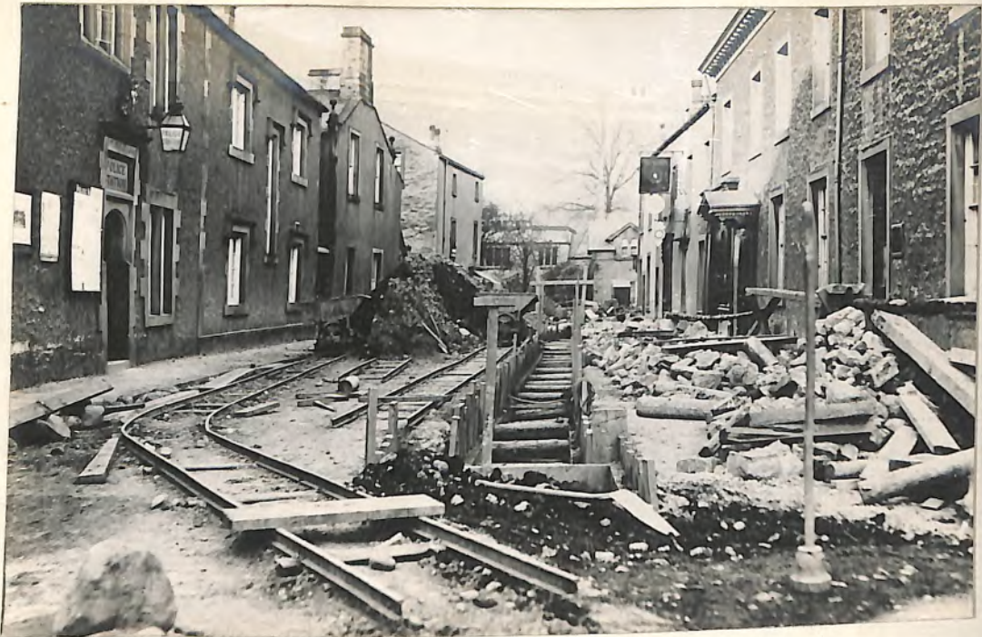
Re-sewering of Settle. New St.
