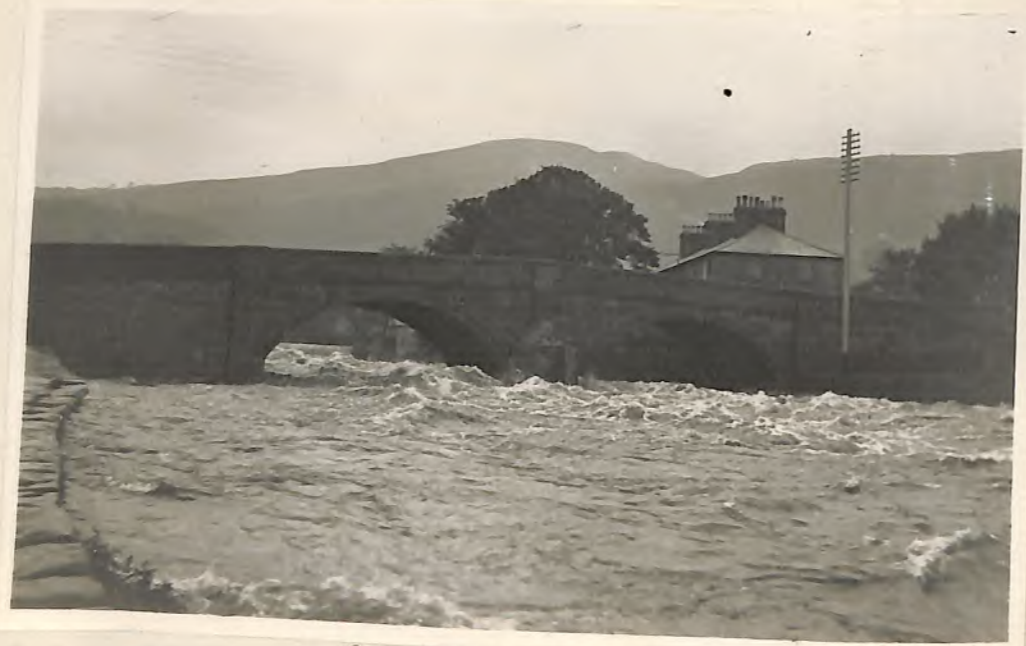
Settle Bridge. 6 Oct 1916.
