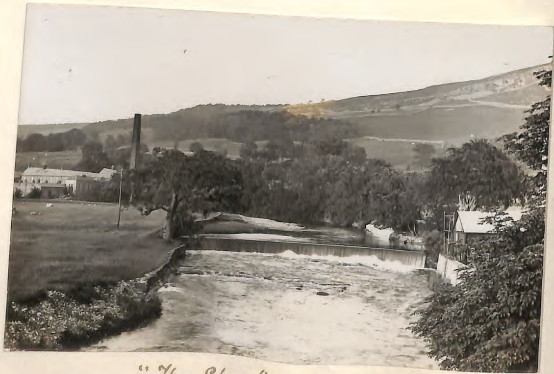
"The Shed", and weir.
