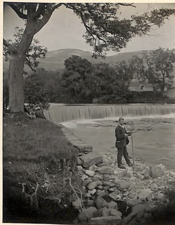
Weir above Settle Bridge
