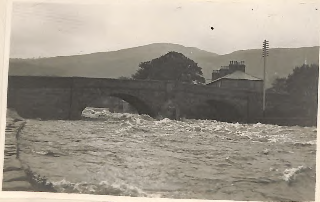
Settle Bridge. 6 Oct 1916.
