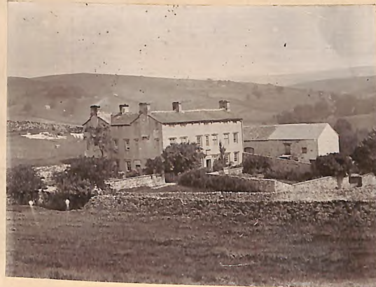
Little Stainforth Hall.
