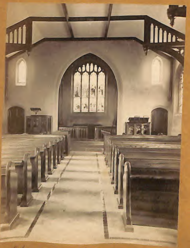
Stainforth Church before restoration.
